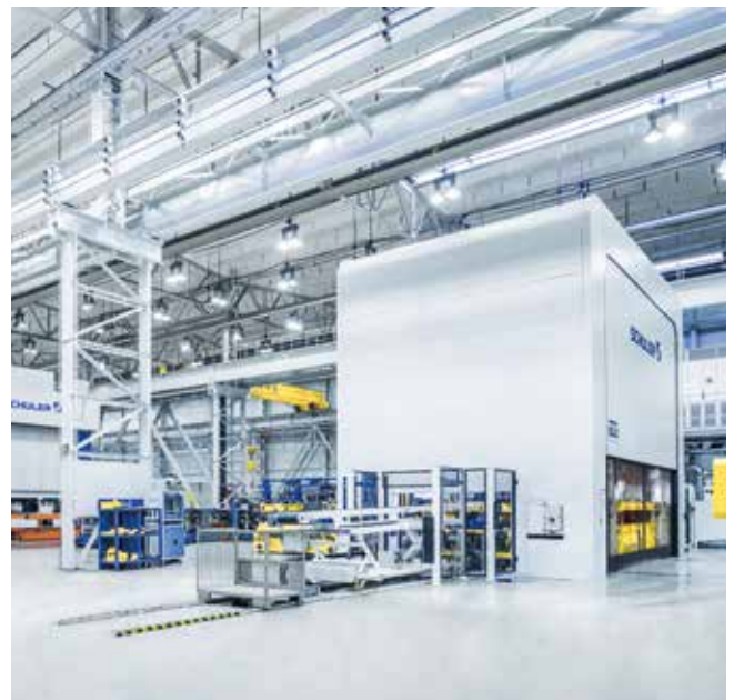
The press plant in Erfurt with three transfer presses.
