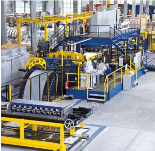
Blanking line with cross-cut shear.
