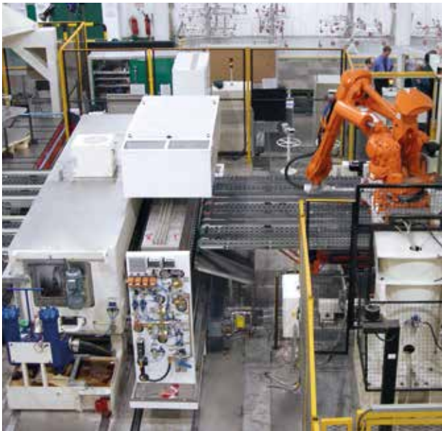
Blank washer, oiler and loading robot in front of hydraulic press line for manufacturing aluminum parts.
