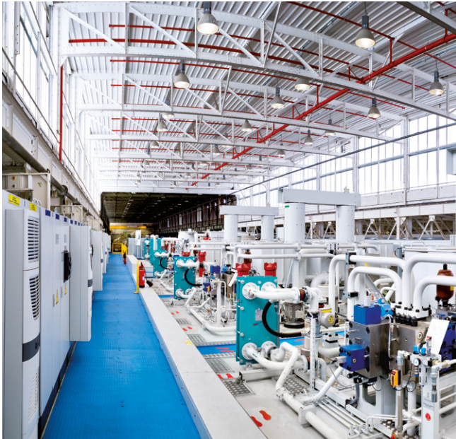
The hydraulics are easily accessible.
