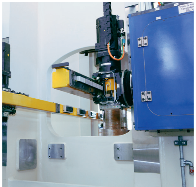
Installation of the transfer in a screw press.
