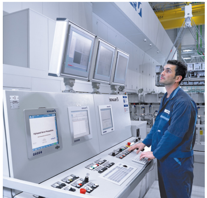
In the control room, the line operator has an overview and control of the complete production process.
