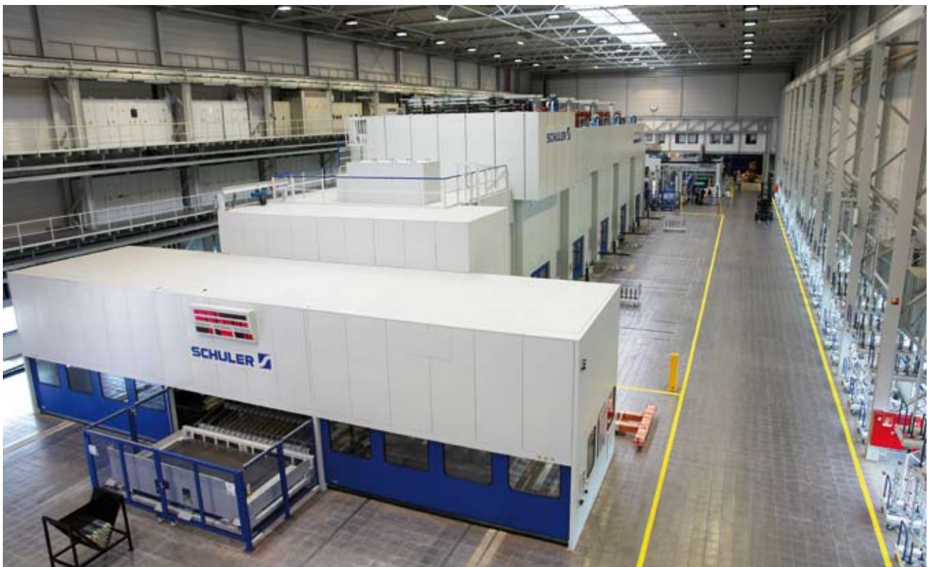
Hydraulic press line with blank loader and robot automation with a total capacity of 89,000 kN.
